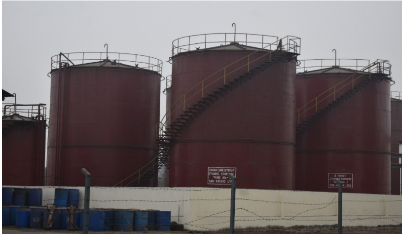
Image: Ethanol storage tanks at Uttam Sugar Mills Ltd.
